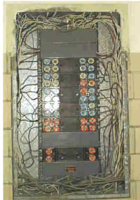
**Figure 6.** Hot neutral wire in an old fuse panel due to undersizing.
