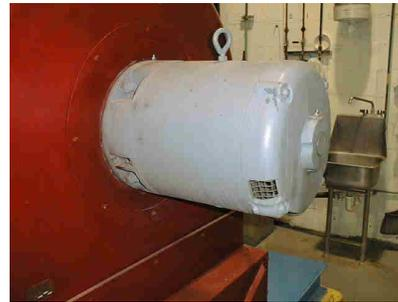
**Figure 7.** Overheated outboard bearing on a 60 HP electric motor driving a boiler blower.
