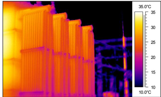
Figure 4d. LN regulator No. 2 radiators after filling
