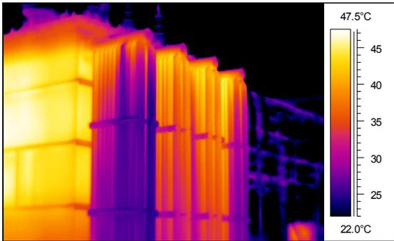
Figure 4c. LN regulator No. 2 radiators before filling
