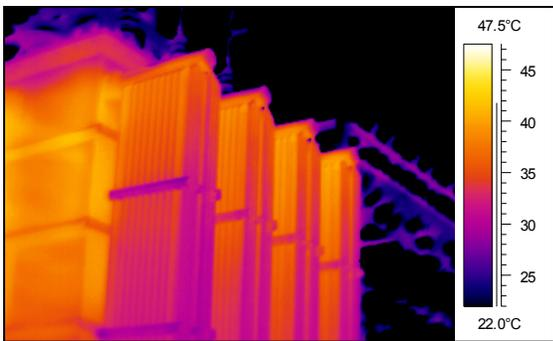
Figure 4e. LN regulator No. 3 radiators before filling
