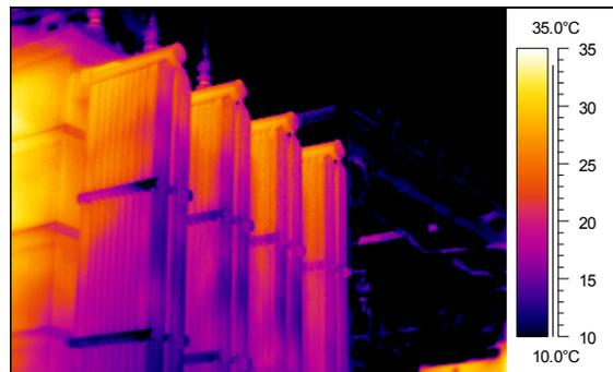
Figure 4f. LN regulator No. 3 radiators after filling
