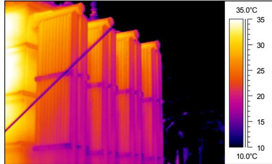
Figure 4b. LN Regulator No. 1 radiators after filling
