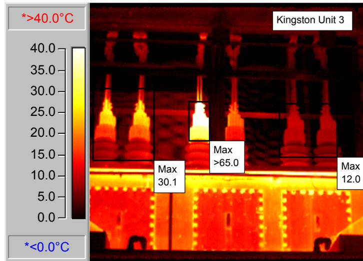
During an infrared scan it was noted that three bushing caps were hot. Bushing caps are rated critical if greater than 35 C rise over another bushing under like conditions. Bushing caps are rated serious if the rise is greater than a 10 C. One had a temperature rise of greater than 53C, which put it in the critical category. An investigation found that aluminum bolts were used instead of stainless steel. Over time the connection became loose, thus creating an overheating condition.
