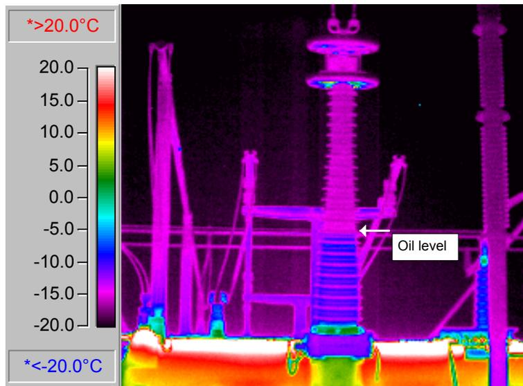
During an infrared scan it was noted that this 500 kV bushing had a low oil level. The oil was leaking from the bottom of the bushing into the tank and was not visible from the outside. The low oil reduced the insulating ability of the bushing. If this had not been found, the bushing would have lost more oil until the point when the insulation would have flashed over. This would have destroyed a 4 million dollar transformer.
